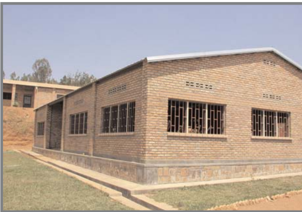
Rwanda Bible School Dining room and kitchen building
